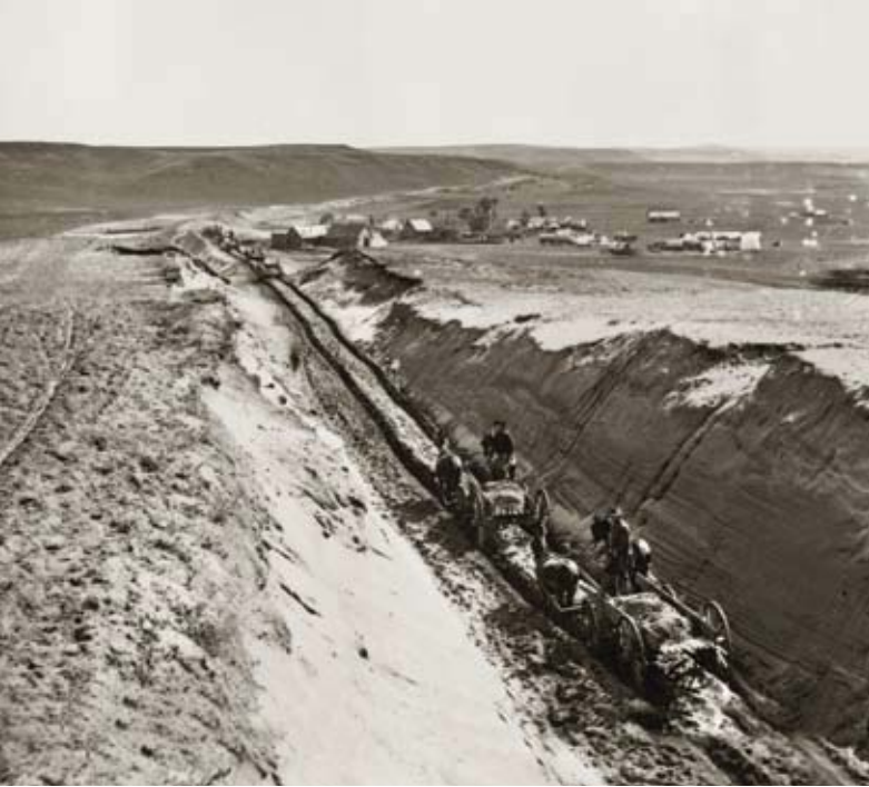
FIGURE 9.5: Laying flat track across uneven territory required dynamite to loosen rock, horse-drawn wagons to move dirt, and endless hours of shoveling by hand.
